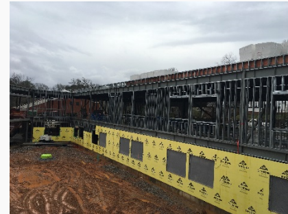
Exterior Sheathing & Framing at Courtyard
