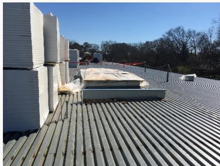
Roof Decking, Insulation, & AHU Curbs
