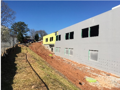
Exterior Sheathing, Air Barrier, & Brick Clips
