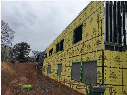
Exterior Sheathing & Air Barrier Prep Work
